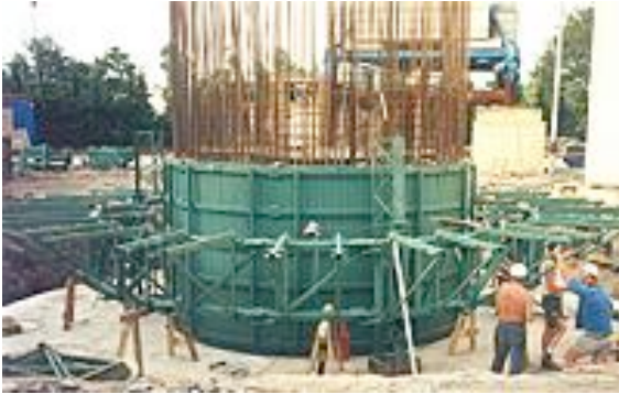
1. Basic assembly of cylindrical formwork and working platform
