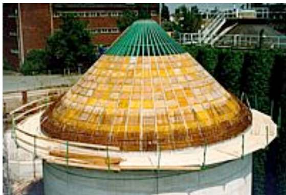
12. Placement of wooden formwork skin
