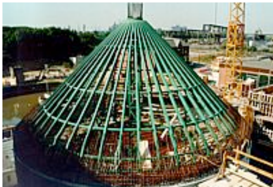
11. Supporting steel structure of the conical roof formwork assembled
