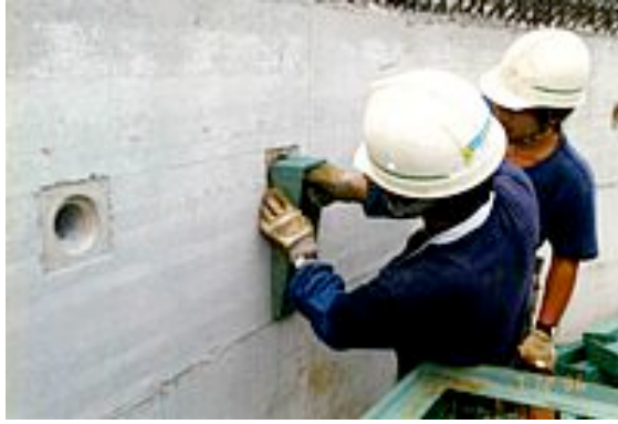
9. Assembling the support ring for the conical roof formwork
