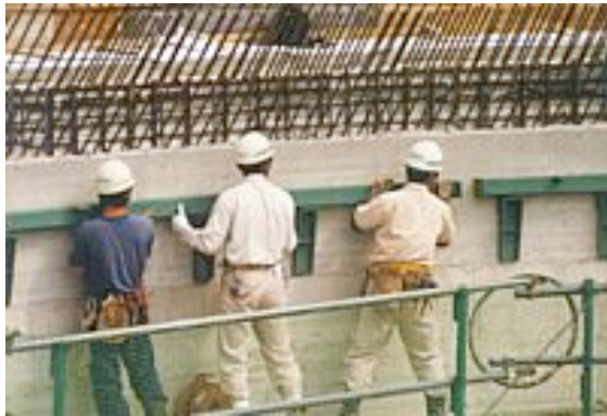
10. Assembling the support ring for the conical roof formwork
