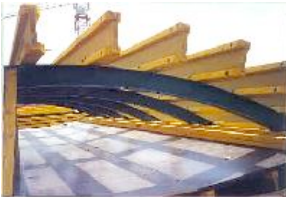
Precurved special formwork for baffles
