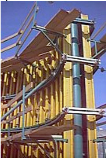
Circular formwork for baffles
