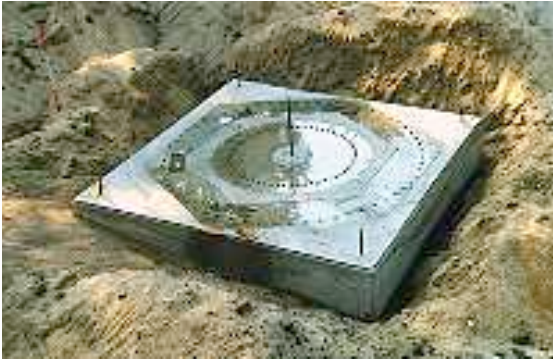
Uplift protection to tie the funnel-shaped formwork
