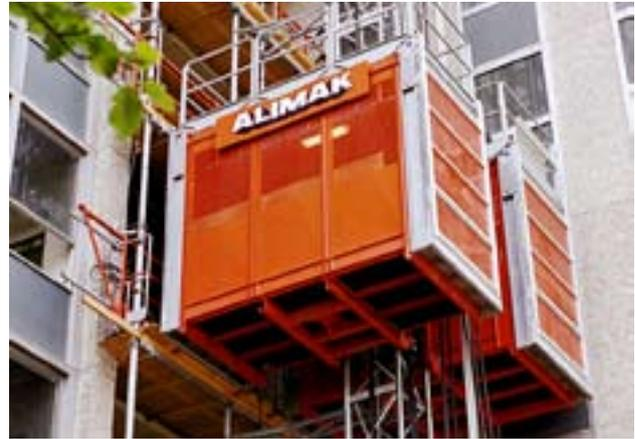
Access is provided by a dual-car Alimak Scando 650 19/32 FC construction hoist, with a lift speed of 54 m/min. Starting at the top floor, demolition robots are working their way down the building. They are transported down to each floor in turn using the Alimak Scando 650. Demolition materials are handled by compact skid-steer loaders, which are also transported between floors by the hoist.
