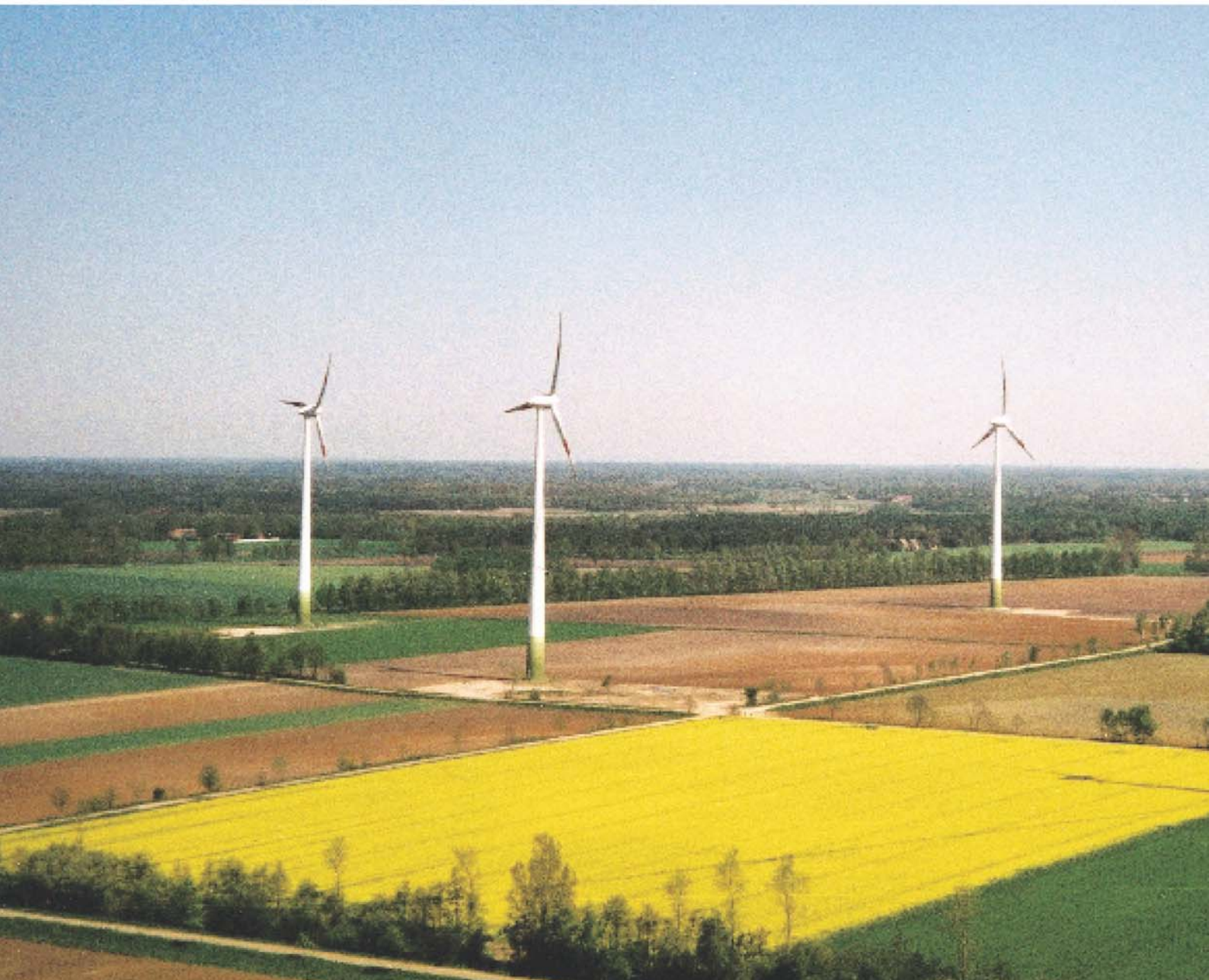
One of two windparks in Meppen, Germany, with 6 windmill towers each, hub height 98 m
