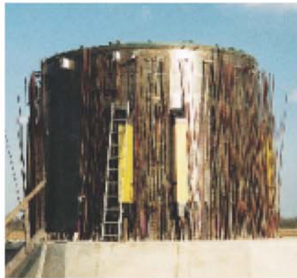
Interior formwork for base section
