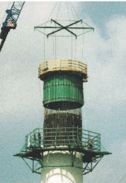
Exterior formwork is lifted in place
