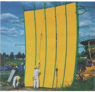
Assembled formwork segment
