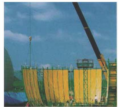
Placing assembled formwork segments
