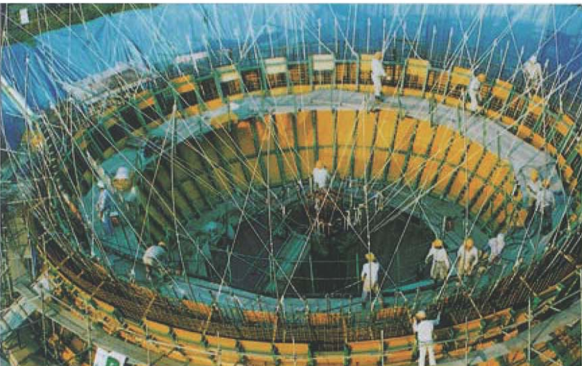
Assembled formwork segment
